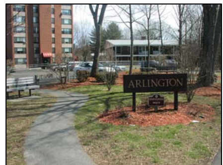
Example Simple Wayside : Bench, Landscaping, Sign
